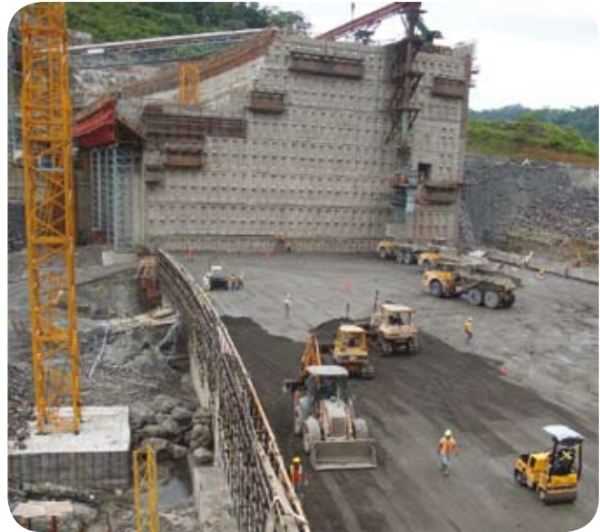
Overview of dam construction (top left), concrete placement on dam (above) and RCC plant (left)
