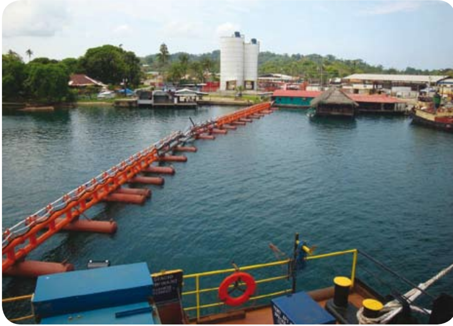
Floating pipeline to silos (above), floating terminal (above right), pneumatic discharge of floating terminal (far right), Indian canoe close to floating terminal (right)
