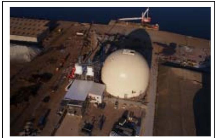
Cement is withdrawn from the dome by means of an Ibau fluidized floor reclaim system which feeds a bucket elevator just outside the dome structure. The bucket elevator is surrounded and supported
