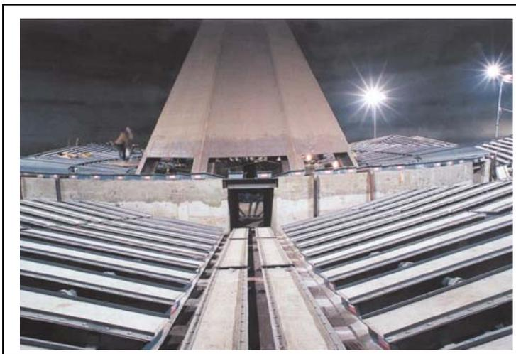
Pneumatic equipment has few moving parts, keeping maintenance costs low. Blower equipment is also minimized by the design for cycling through the various rings and sectors. The energy to operate the system is only about 0.16
