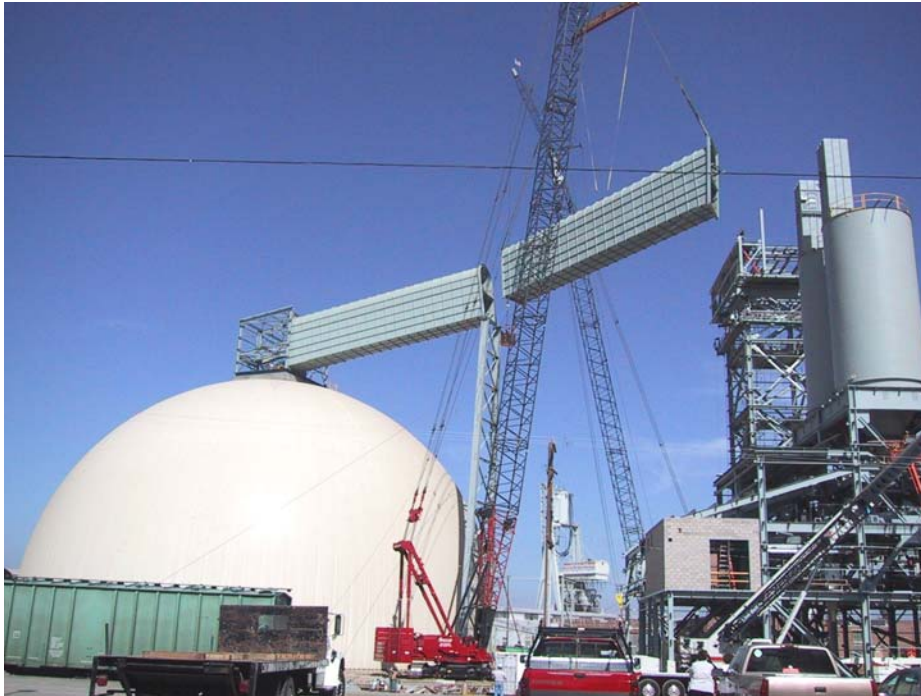
Figure 9 – Installing CamSpan Gallery
