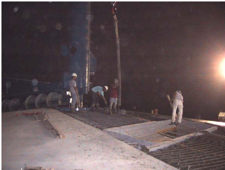
Figure 4 – Construction of Concrete Floor
