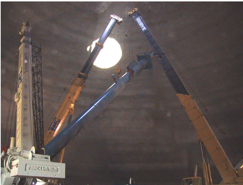
Figure 8 – Installing Reclaim Center Column
