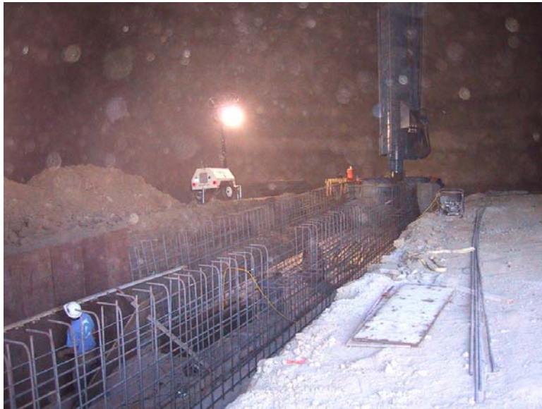
Figure 3 – Air Gravity Conveyor Tunnel under Construction
