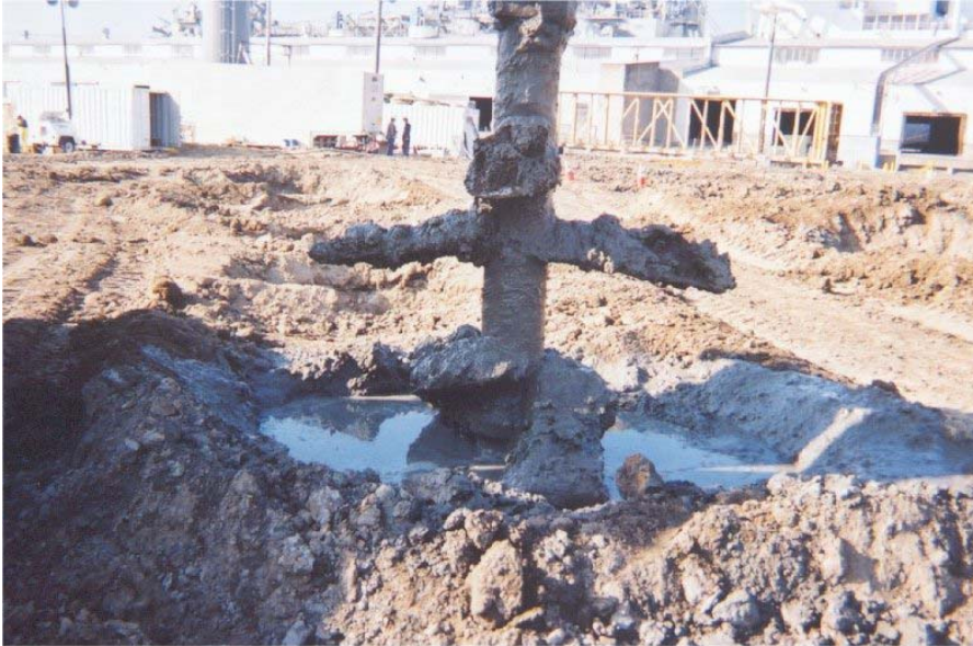
Figure 2 – Soil / Cement Blending Process
